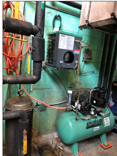
Pneumatic compressor serving HVAC controls.
