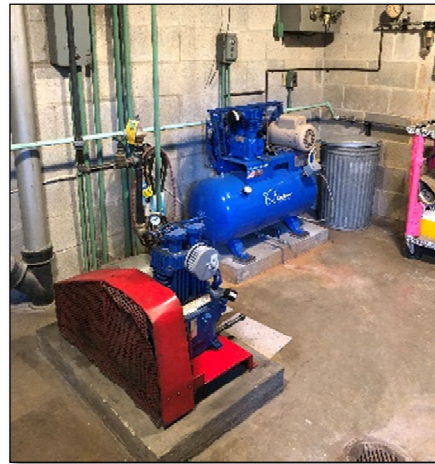
Pneumatic compressors for HVAC controls and drinking fountains.
