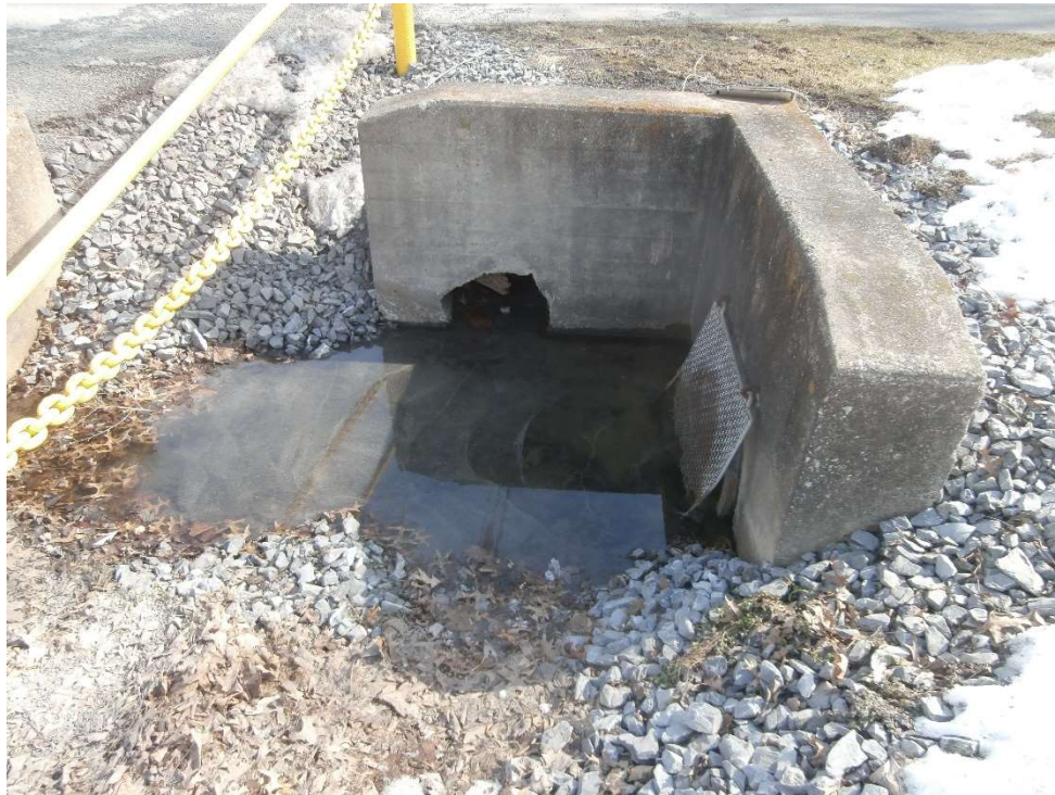
Figure A18: The culvert (straight ahead) appears to be deteriorating as shown by corrugated metal hanging from what should be the top of the pipe. The trash rack on the other pipe opening (right) is deteriorated and detached from the endwall structure.
