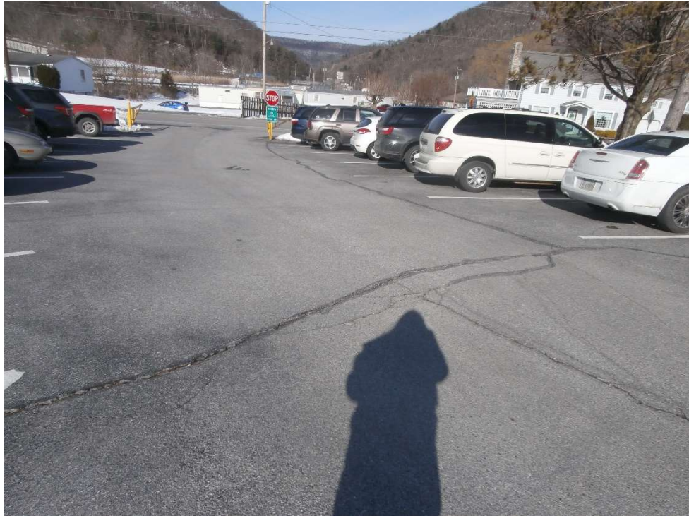
Figure B3: Deep cracks exist throughout the parking lot.
