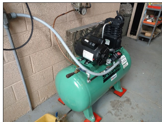
Air compressor for Pneumatic HVAC controls.
