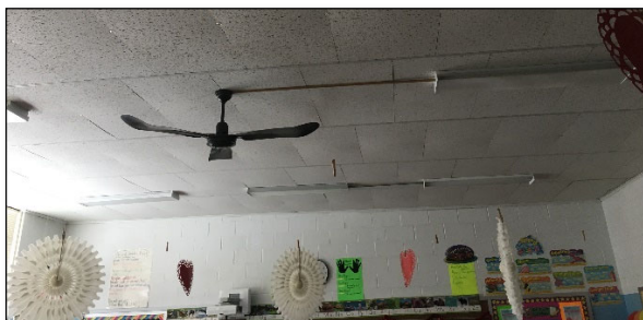
Classroom lighting consist of 1'x4', ceiling mounted, 2-lamp 32-Watt T8 lamps, fixtures.
