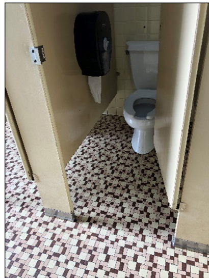
Toilet's china is in good condition but are high flow fixtures.
