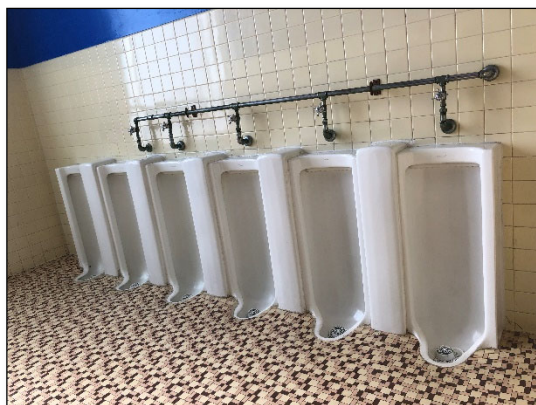
Floor mounted urinals have on/off fixtures.
