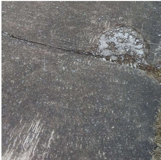
Figure D6: There are areas of damaged concrete along the front of the school.
