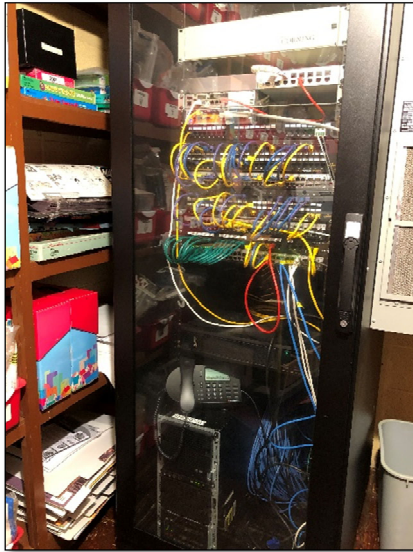
Server is located inside the MDF book room. Thermal Edge Inc, model NE08012612, R422d.
