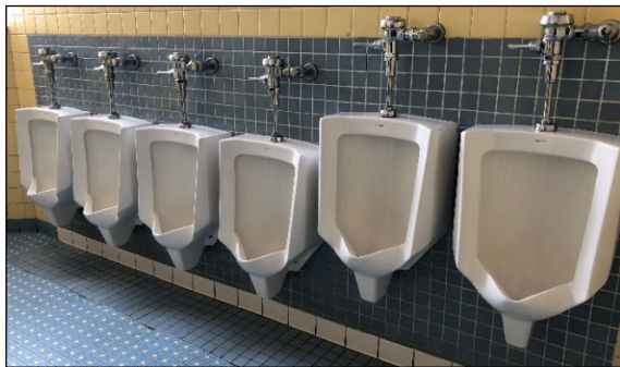
Urinals are in good and serviceable condition; however these are high flow fixtures (3 GPF).
