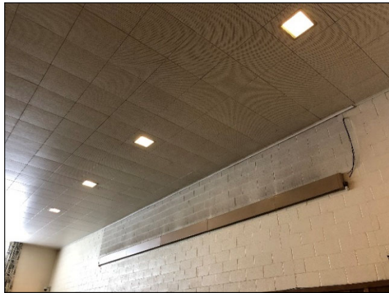
Steam radiators in the multipurpose room.
