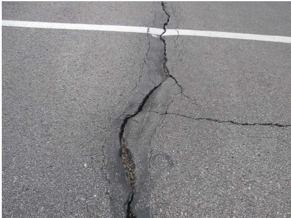
Figure A12: In some areas of the asphalt playground, cracks are very deep and wide. This portion of the crack has been sealed before.
