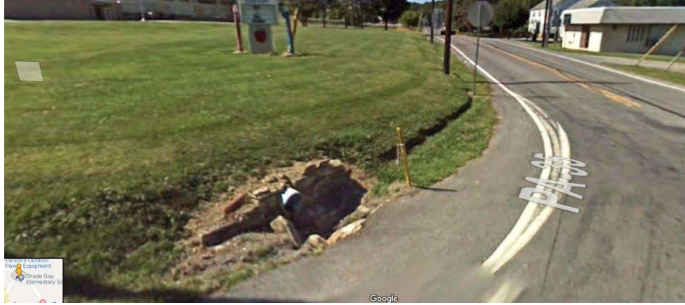
Figure B9: The pipe at the intersection of PA Route 35 and PA Route 641 appears as though it could have a drainage problem at this pipe discharge. This was not observed while on site, but rather on Google Street View.
