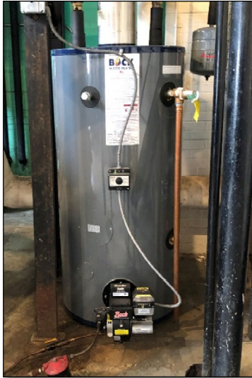
Domestic water heater: Bock, model 72E, installed in April 2017. Capacity: 199 MBtuh, 68 gallons.
