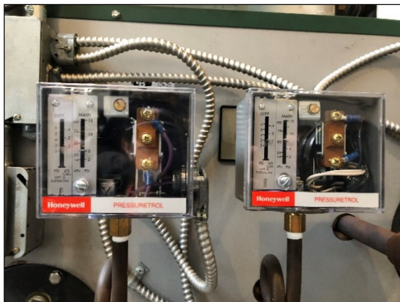
Boiler controls setpoints: Difference pressure 3 PSI; main at 5 and 7.5 PSI.
