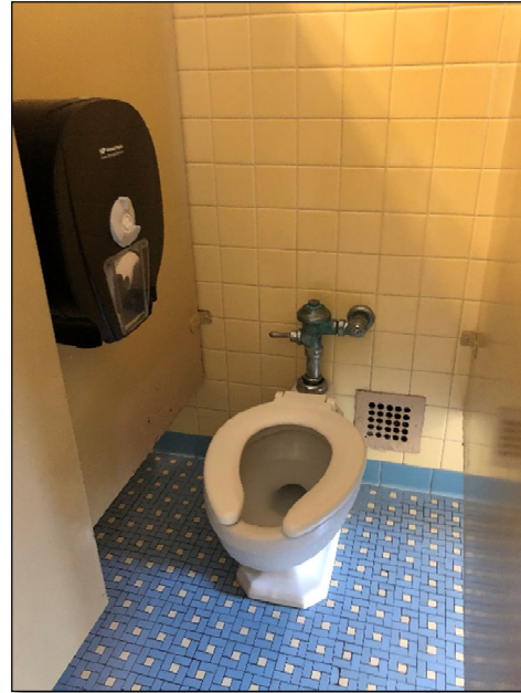
Toilets are high flow fixtures (3.5 GPF).
