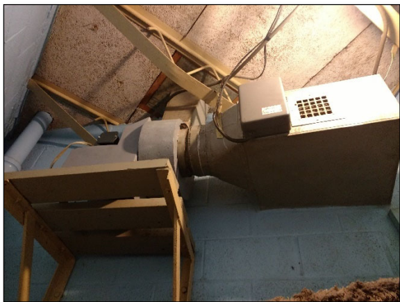
Bathroom exhaust fan.
