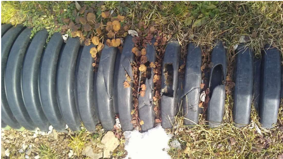
Figure D20: The outlet pipe located near the baseball field is uncovered at the top, and is damaged.
