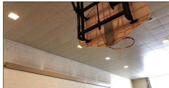
Multipurpose room lighting consists of HID recessed cans.
