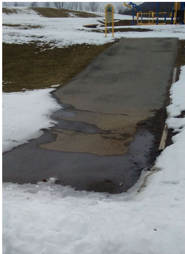
Figure C4: The ramp leading to the playground does not appear to be ADA compliant in terms of slope.
