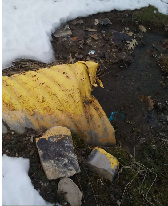
Figure D13: A culvert pipe near the Coulter School is deteriorated and damaged.
