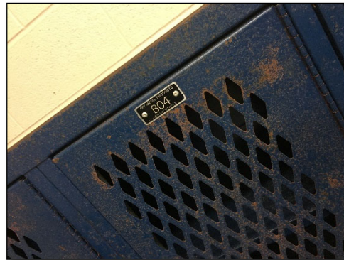
Humidity in locker room has rusted the lockers. They need to be re-painted.
