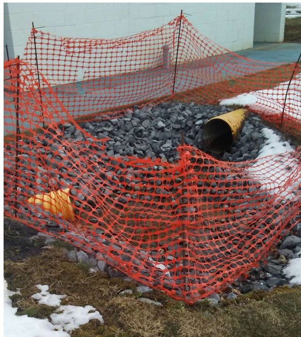
Figure D18: According to Stanley Hall, this fencing was erected at the end of the 2018 football season as a result of a washout. Hall indicated that he intends to make this a junction point with a grate over top.
