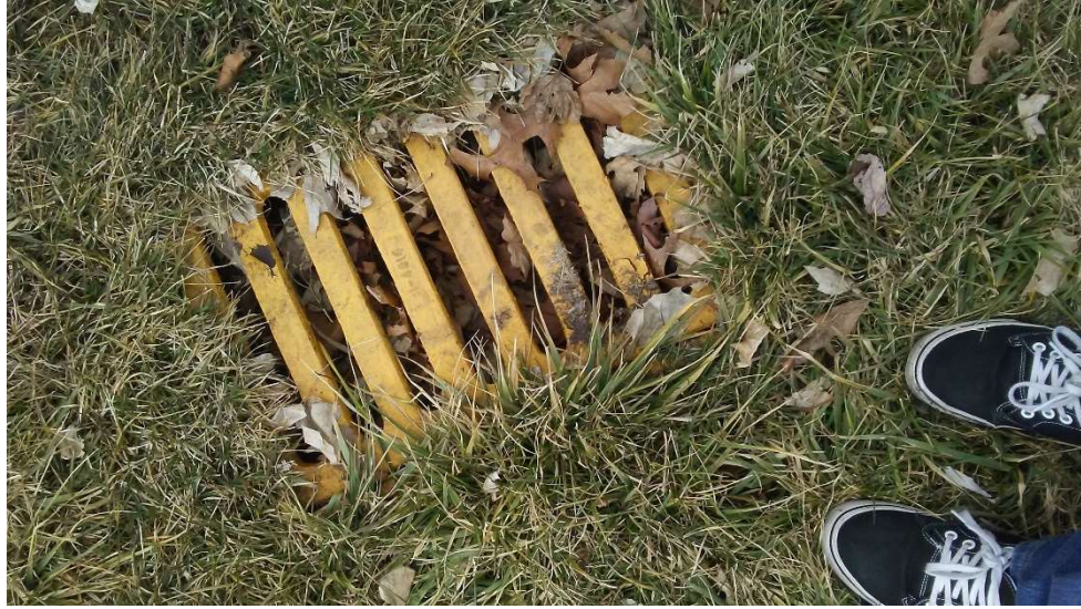
Figure C11: The inlet appears to be full of debris and should be cleaned.
