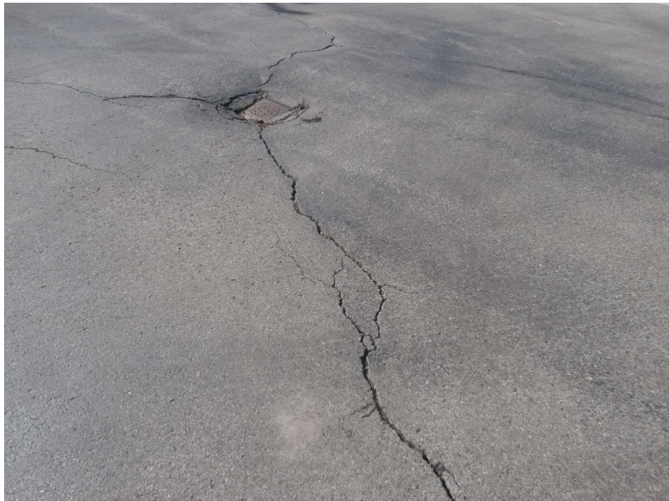
Figure A20: The structure in the middle of the asphalt play area appears to have caused cracking in the pavement that extends radially outward from the structure.
