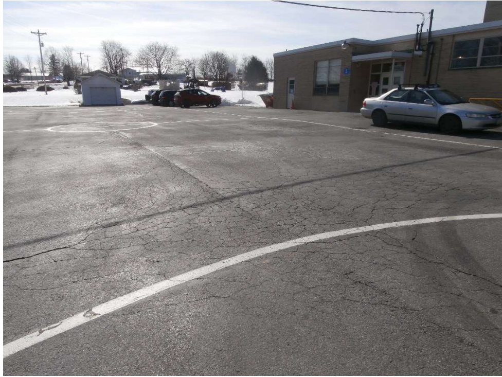
Figure B5: Typical alligator cracking on the eastern side of the school.
