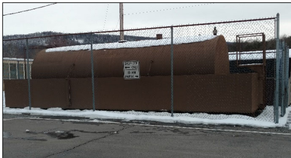
10,000 gal fuel oil tank above ground. 25 years old.
