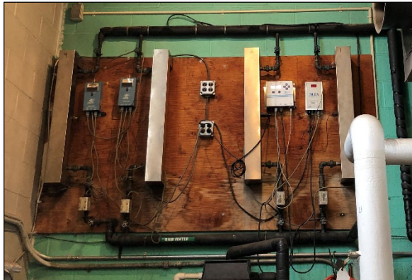
UV light purification system for domestic water.
