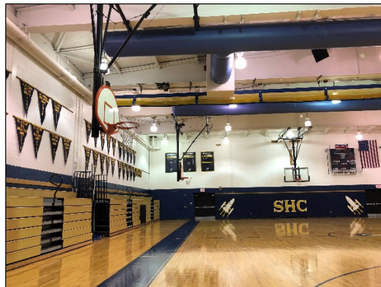
Gym lighting consist of 30 metal halide fixtures. Auxiliary gym also has 20 metal halide fixtures. Lighting is generally in good condition but given the technology and increased hours of operation of these areas for community use, LED technology should have a good payback.
