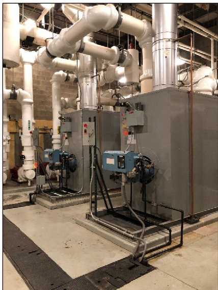
2 Boilers provide heating hot water to the site. Manufacturer: Ryan Boilers. Model RV400 W FDO, built in 2003. No need for improvements.
