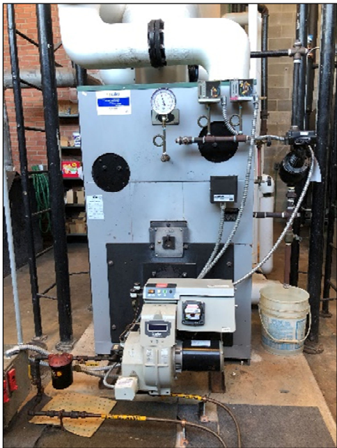
Boiler: Peerless Boilers, model LCE-13 W/S. Capacity 2,464 MBH. Gross output 1,966 MBH steam. Burner R. W. Beckett Corp., model CF2300A. Firing range: 7-19.9 GPH.
