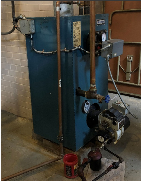
DHW Heater: Burnham Corporation. Model RSA135TH-TB, 156 MBH (2002). Coupled with Weil McLain hot water tank; model PLUS 120, 120 Gal.
