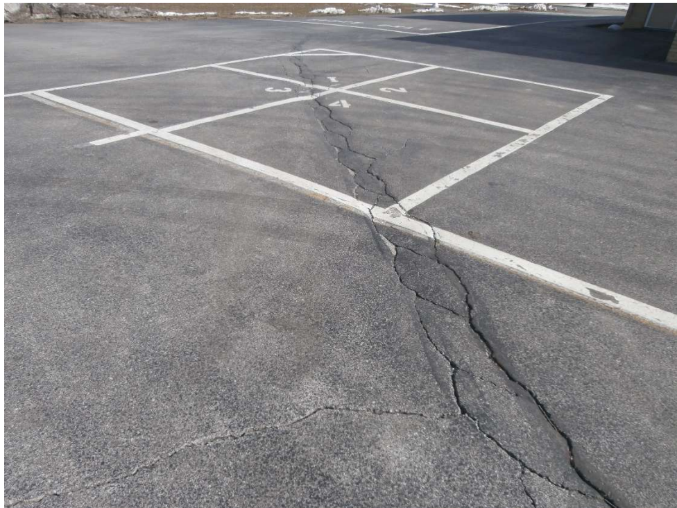
Figure A14: The play area at the side of the school appears to be subsiding at what could be the location of piping.
