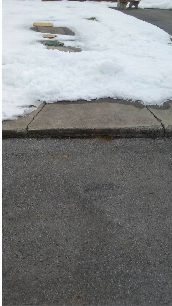
Figure C5: Pavement at the play area appears to have sunk, creating a tripping hazard with the connection to the sidewalk.
