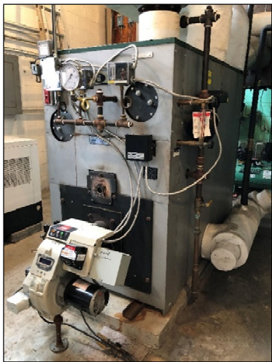
Steam boiler Peerless Boilers: LC-12-W/S. 15.6 Gal/Hr Oil; serial No. 630047-200911; IBR 1,593,000 Btuh Steam (2010). Burner: Beckett Model CF2300A.
