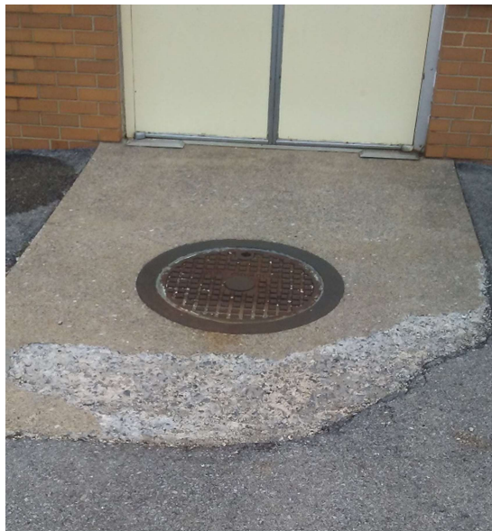
Figure C8: The concrete slab has been damaged.
