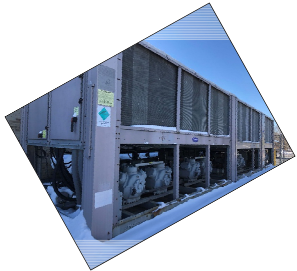
2 Carrier air cooled chillers provide chilled water to the site.
