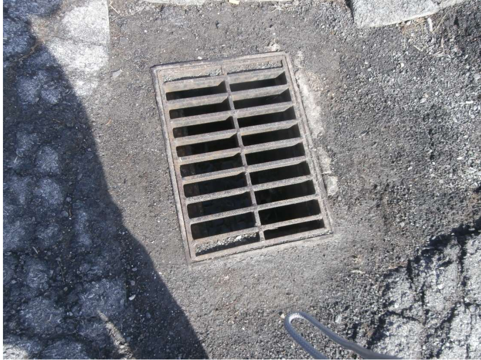
Figure A19: An inlet in the parking lot is surrounded by deteriorated paving.
