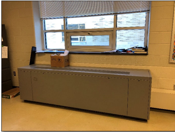
The school has a 2-pipe HVAC system. Most classrooms have a CHW/HW unit ventilator. The system operates in either heating mode or cooling mode.
