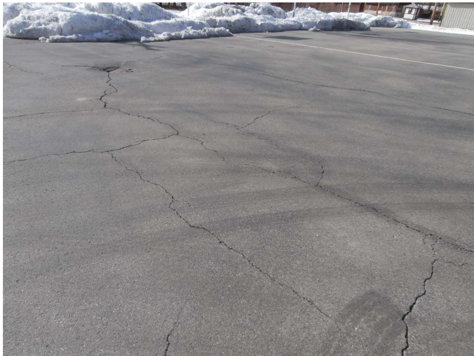
Figure A10: The paved play area shows many cracks.
