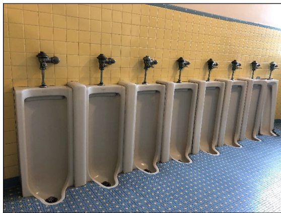
Floor mounted urinals, china is in good condition, however these are high flow fixtures.
