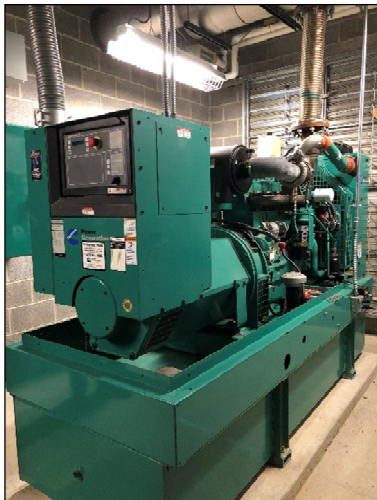
Back-up power generator for emergency loads. Cummins Power Generation, model DGFC-5618999 60Hz/ 13kW @ 1PH, 200 kW@ 3PH.
