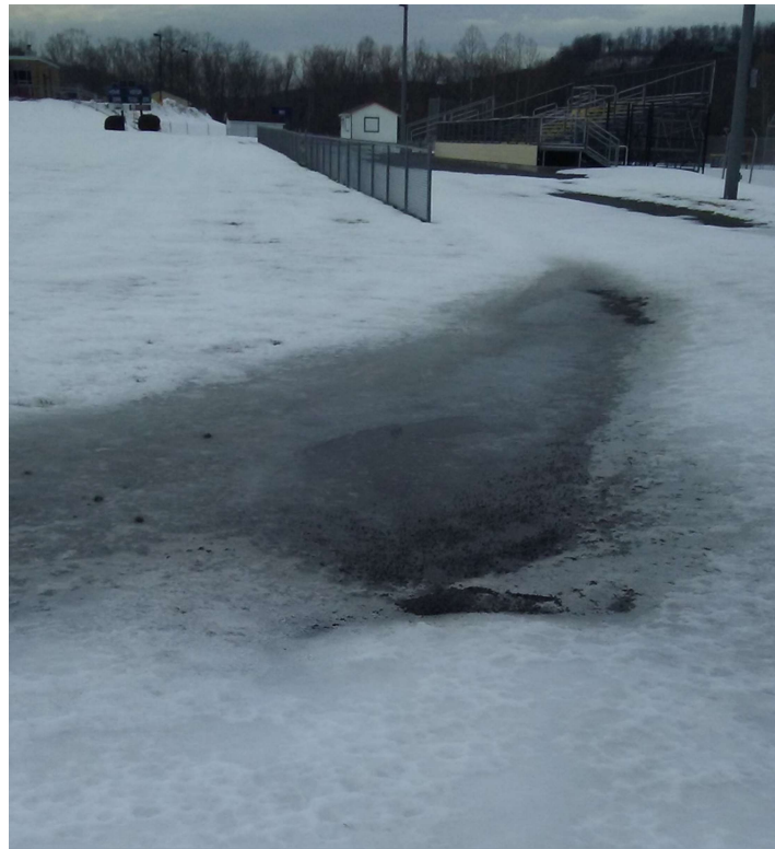
Figure D16: The northeast end of the football field and track appears to have significant ponding, probably due to the grading issue throughout the stadium.
