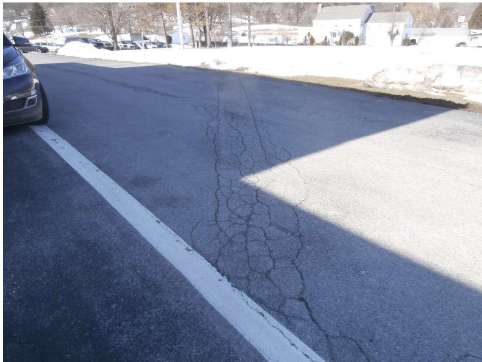
Figure B6: Pavement appears to be subsiding above a pipe leading to the grease trap on site.
