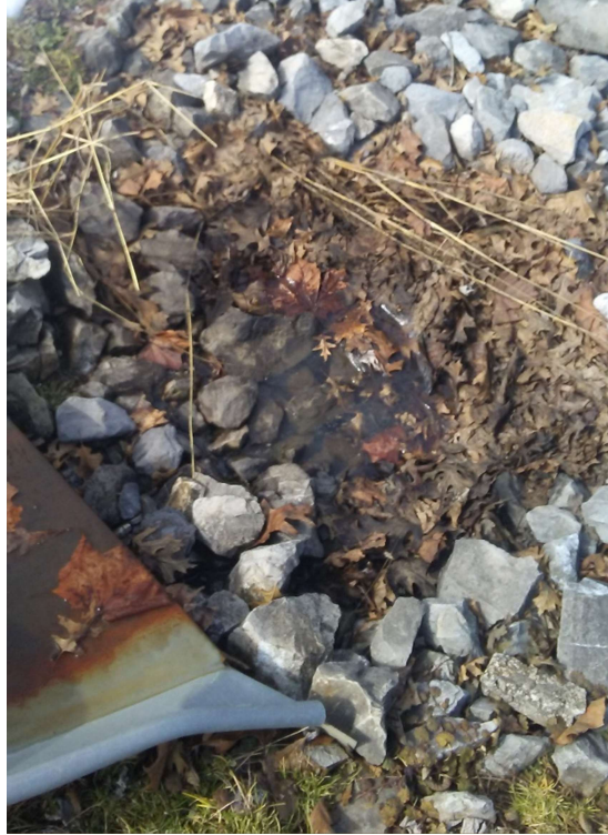
Figure D21: The flared end section drains to a riprap apron that has appeared to wash out, which would result in ponding at this location.
