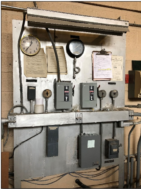
Water Heater, Boiler and Light electric disconnect switches.
