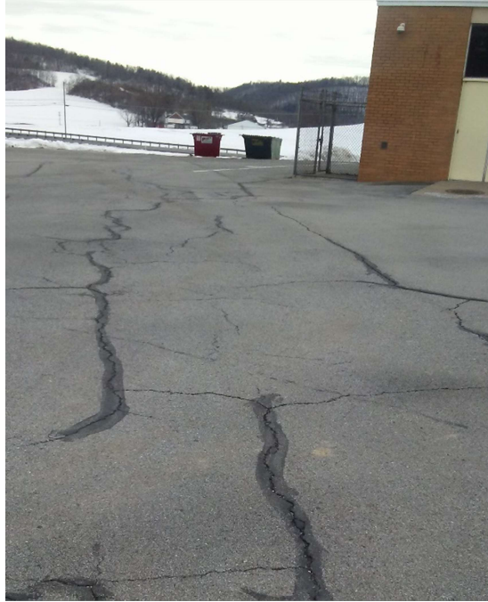
Figure C9: The asphalt play area shows a lot of cracks propagating into other cracks.
