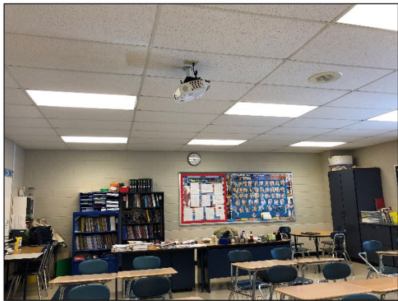
Classroom lighting consist of recessed 2'x4' – 4 lamp T8-32Watt fixtures. Lighting is generally in good condition.
