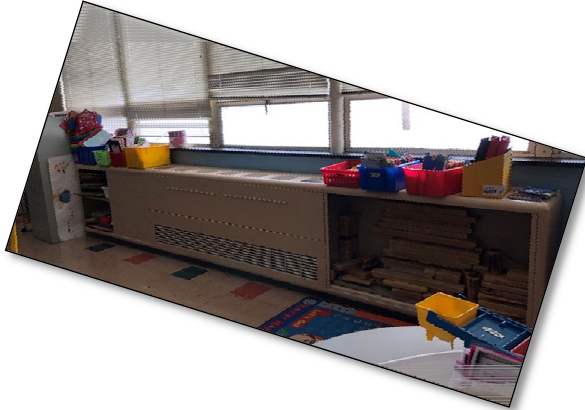
Classrooms are equipped with unit ventilators with fin tube elements.
