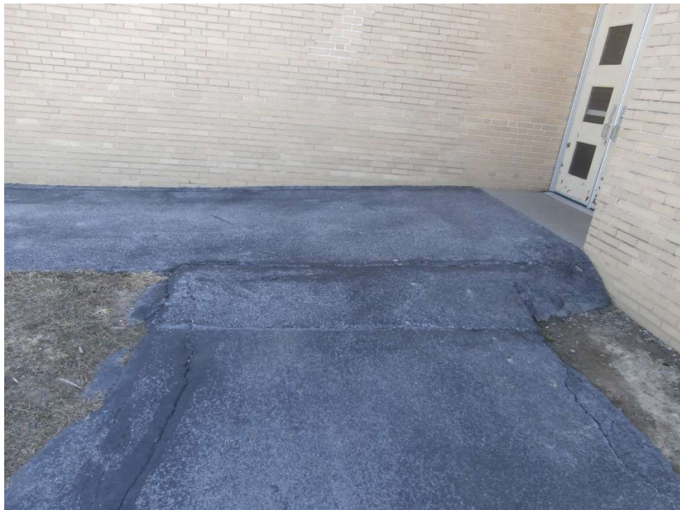
Figure B2: The ramp on the western side of the school building (both leading to the building and to the asphalt path) do not appear to be ADA compliant in terms of slope.
