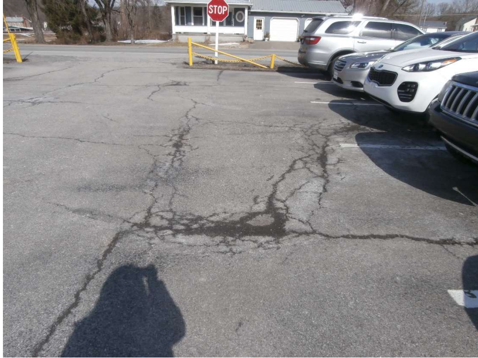
Figure A13: The parking area exhibits alligator cracking.
