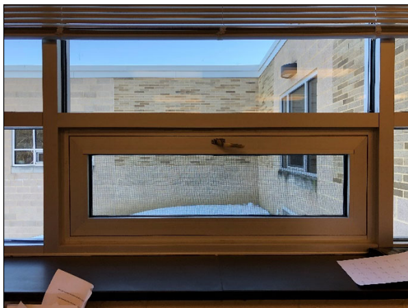
Windows are double pane, with an operable panel. They are in good conditions.
