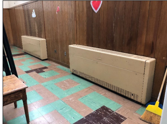
Unit ventilators at the multipurpose room, operate with fans off, except for inclement winter weather.
