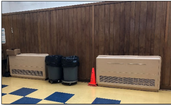
Unit ventilators in multipurpose room are operated with fans off, except during extreme winter weater.
