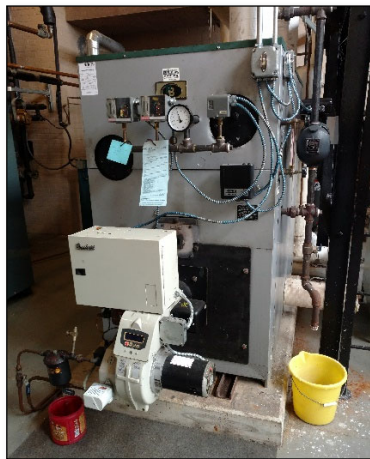
Single low-pressure steam boiler. Peerless Boilers: LC-12-W/S. Serial No 577122-200707, 15.6 Gal/Hr Oil. IBR 1,420 MBtuh. Manufactured in 2007. Burner: Beckett, model CF2300A.
