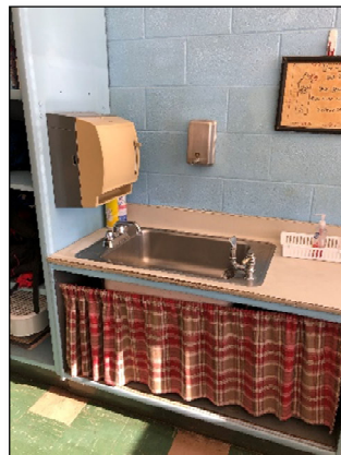
Classroom have individual sinks. Door cabinets failed and replaced with curtains.
