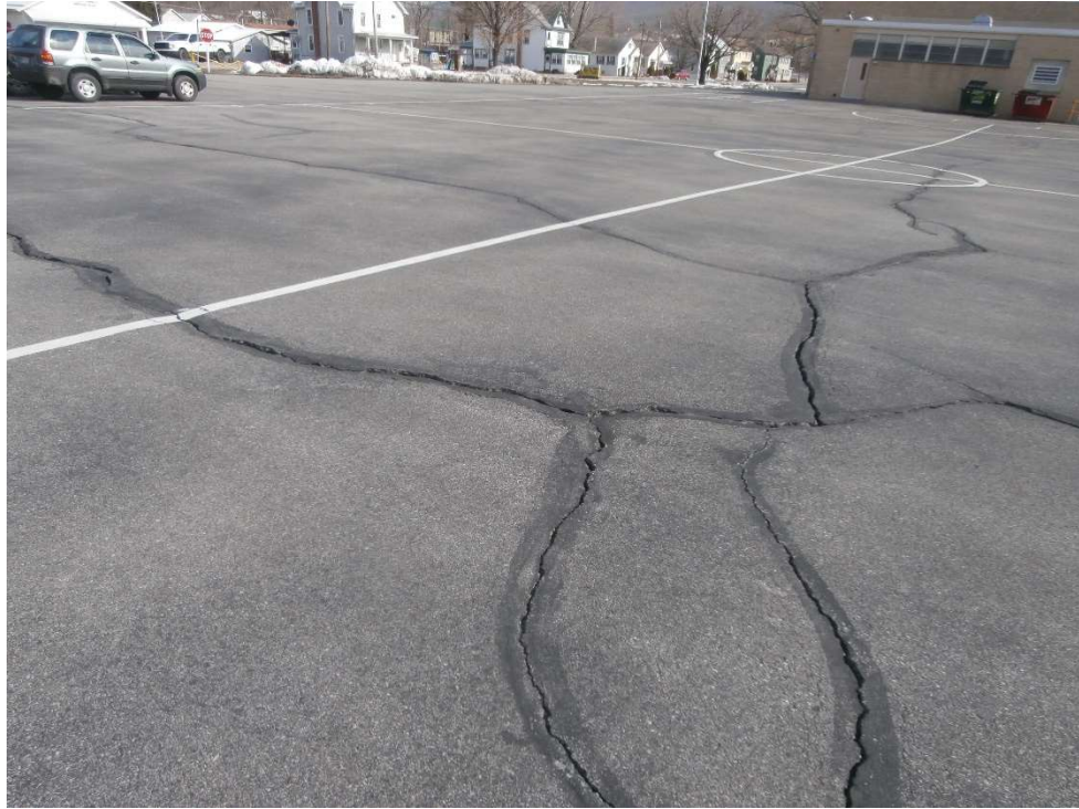
Figure A11: The paved play area shows many cracks.
