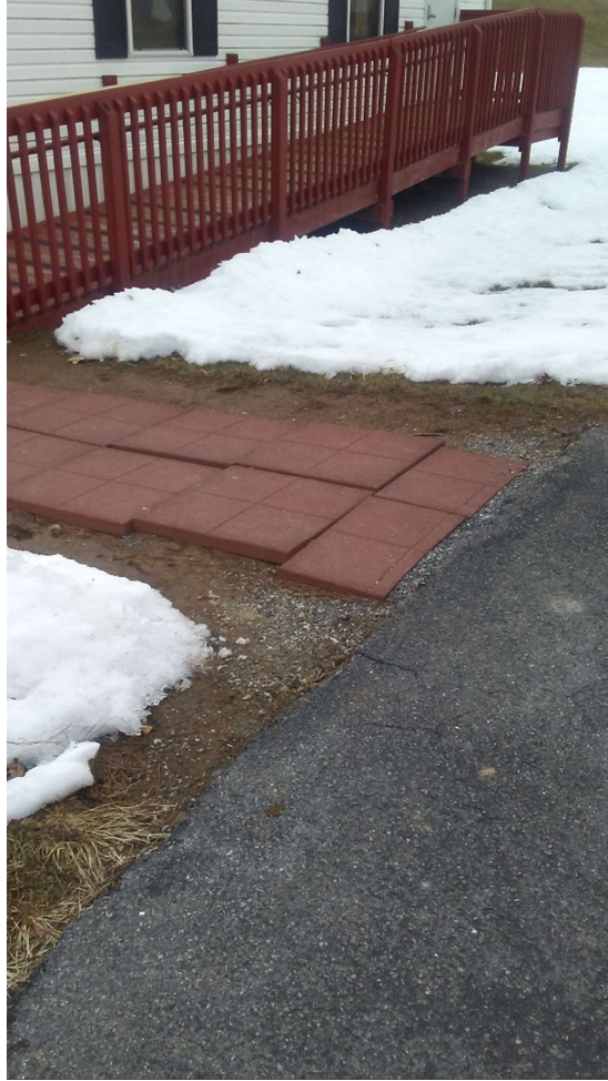
Figure C6: Pavers leading to the modular unit are not level, and create a tripping hazard..
