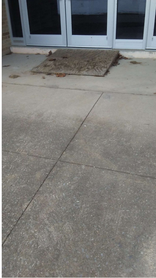
Figure D4: A ramp leading to the front entrance of the building has a plywood ramp.
