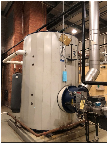
Domestic hot water is produced and stored in a PVI heater.
