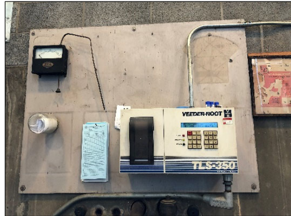
Veeder-Root TLS-350 automatic tank gauge.
