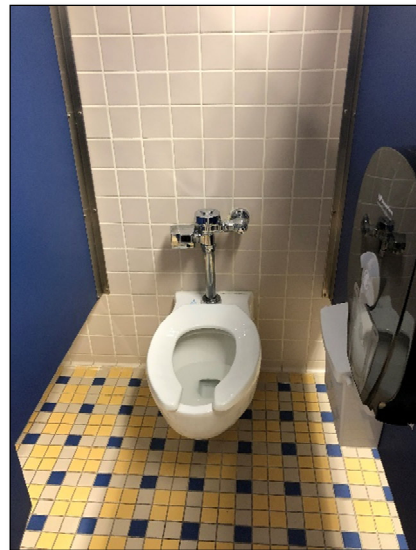
Wall mounted toilets with automatic flush valves.
