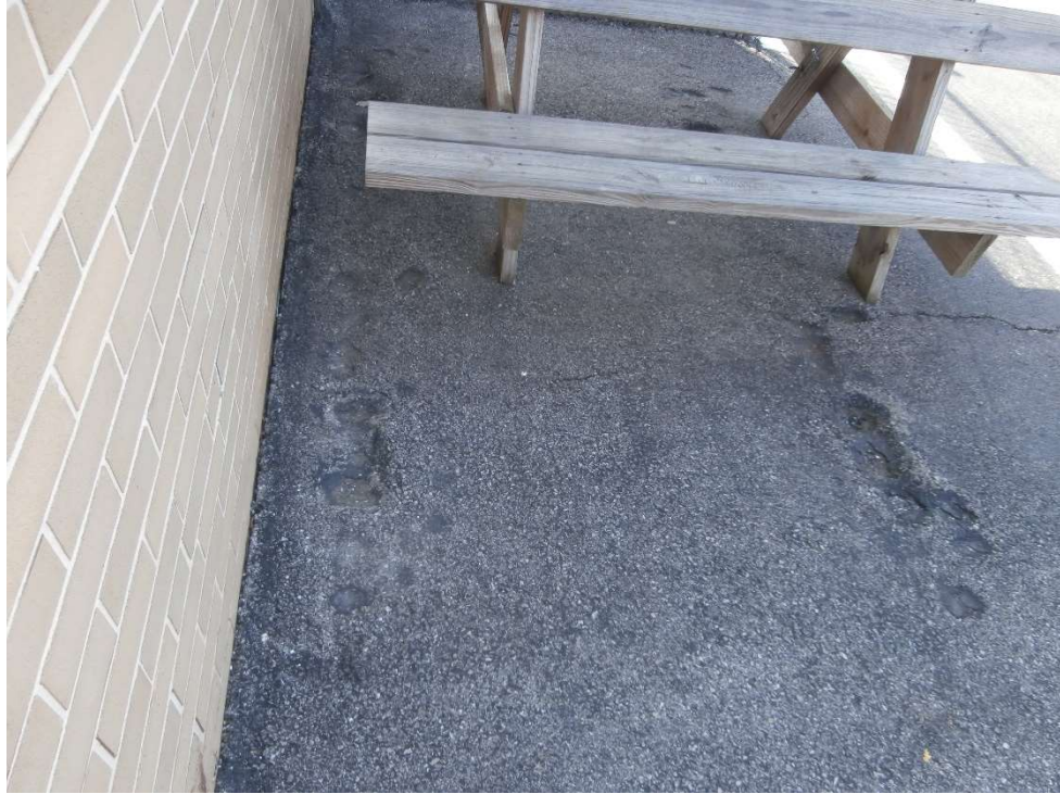
Figure A9: The pavement near the picnic tables shows defects consisting of divets.
