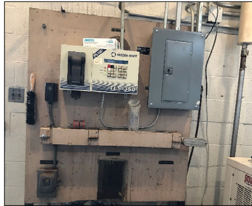
Electrical panels are old and in need of replacement.
