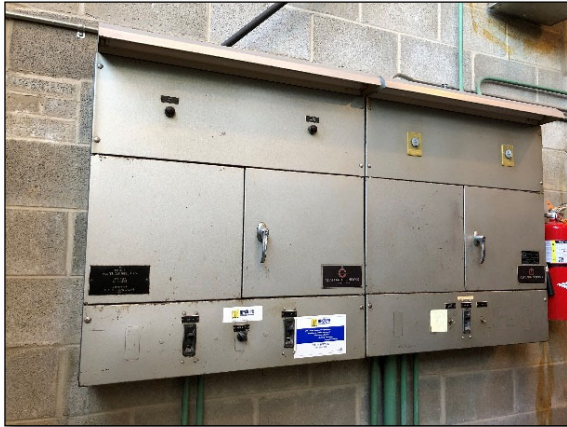
Main electrical panel, original to the building.
