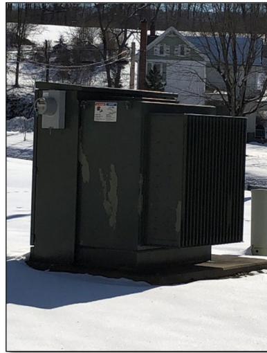
Main power transformer sits outside the school; it is in good condition.
