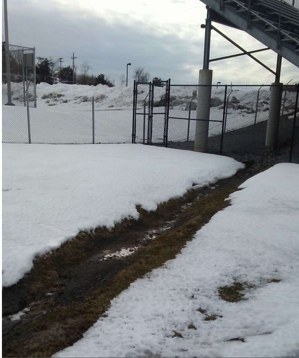
Figure D17: It appears as though this drainage channel was formed as a result of a erosion, which is consistent with conversations with Stanley Hall about the picture below.
