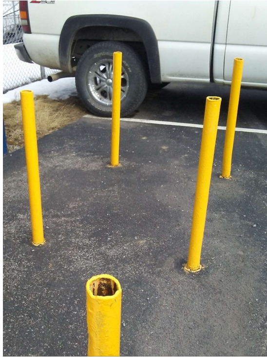
Figure D5: Typical bollards on the site are open pipes at the top, which could be a safety hazard. These are located at the stadium ticket stand, but there are more along the access drive.
