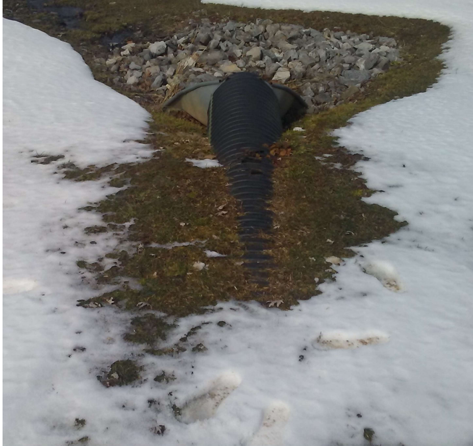
Figure D19: The outlet pipe located near the baseball field is uncovered at the top, and is damaged (see center of pipe).
