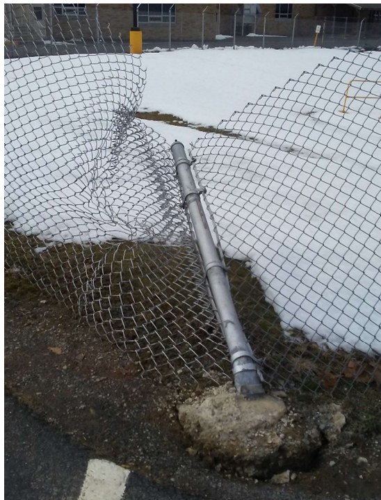
Figure D8: The fence and pole are damaged near the entrance to the football stadium.
