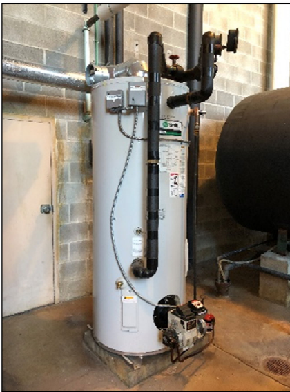
DWH A. O. Smith Water Products Co., model COF 199 940, serial number 1410M000289, capacity 199,000 BTUH, fuel oil, coupled with a HW storage tank w/ water treatment.
