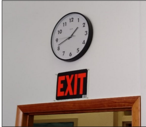
Exit signs are not illuminated but fluorescent stickers.
