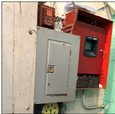
Fire alarm panel and fuses.
