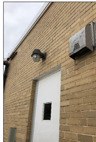
Exterior lighting consist of HID bulbs.
