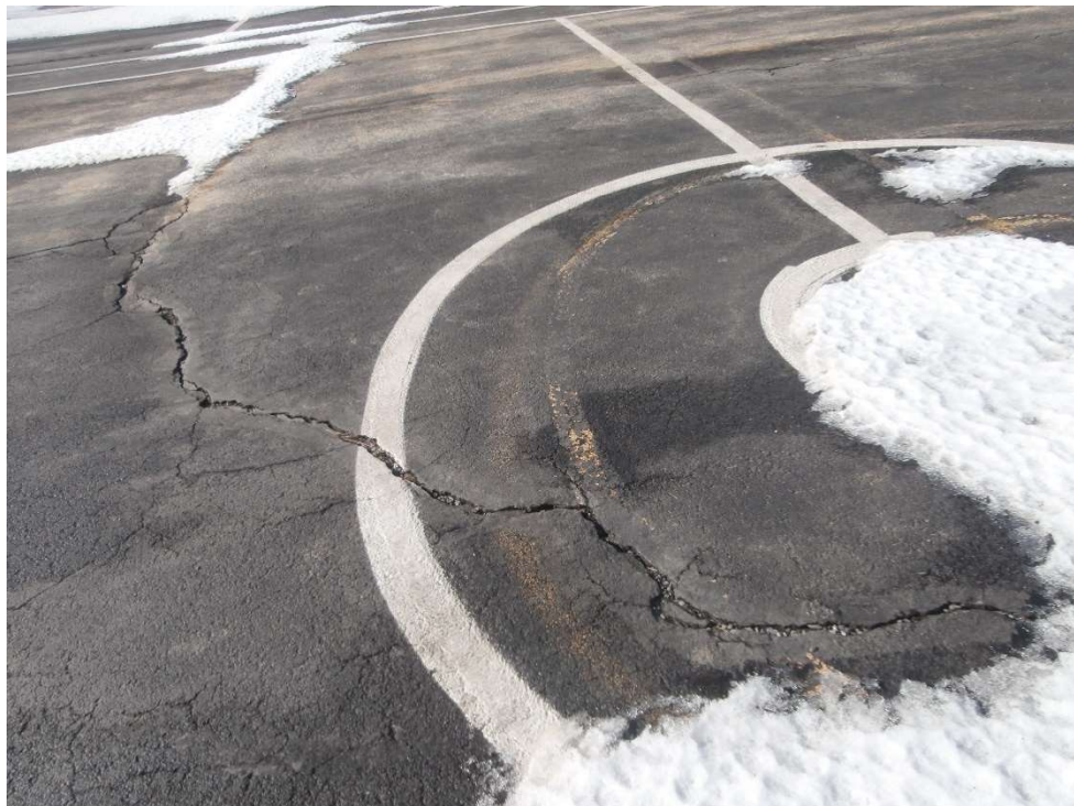
Figure B4: Deep cracks exist throughout the asphalt play area on the western side of the school.
